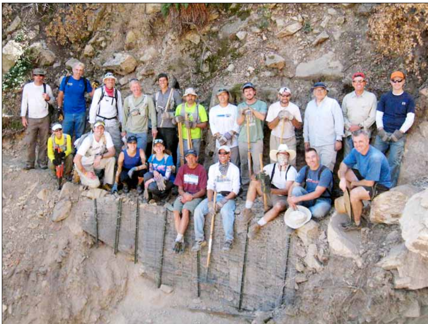
Idle Hour Trail, after repair. Idle Hour trail work, summer 2010. Photos by Hal Winton
