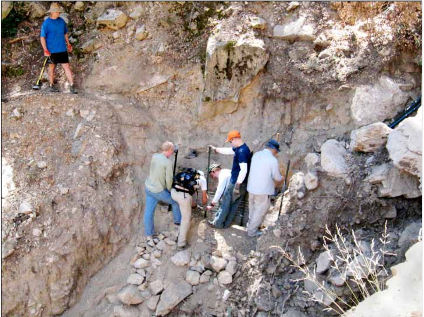
Idle Hour Trail, before repair. Idle Hour trail work, summer 2010. photo by Hal Winton
