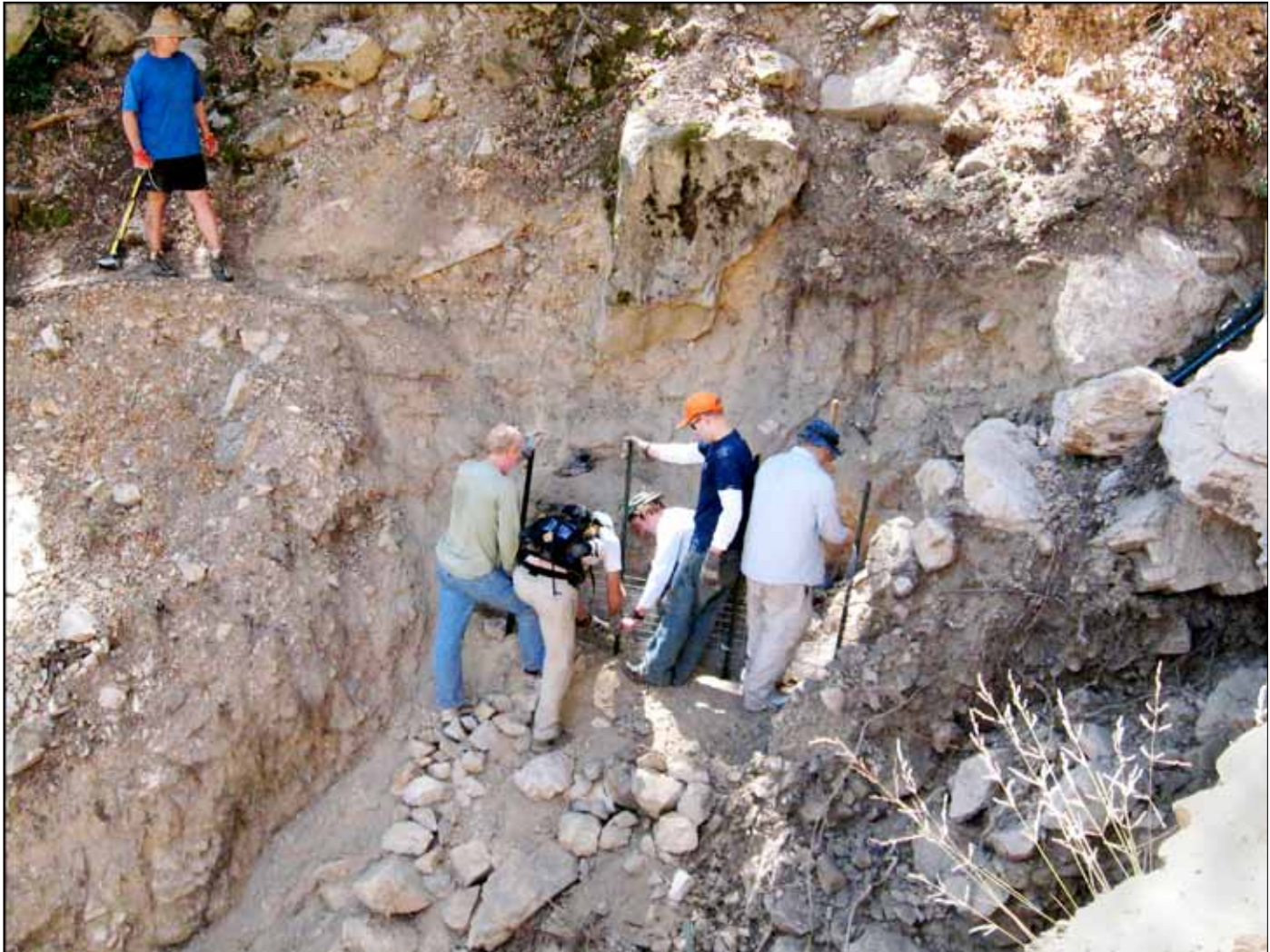
Idle Hour Trail, before repair. Idle Hour trail work, summer 2010. Scott Mills, SD100 RD is on the left in the hole with BSA leader Rich Hoesley etc. photo by Hal Winton
